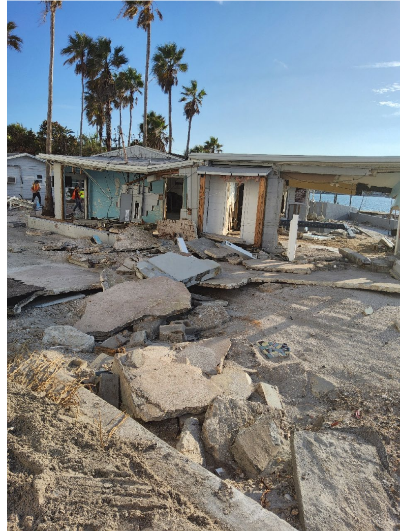
Pass-A-Grille Beach with buildings destroyed and erosion condition IV, near R-166
