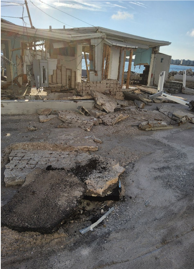
Pass-A-Grille Beach with buildings destroyed and erosion condition IV, near R-166
